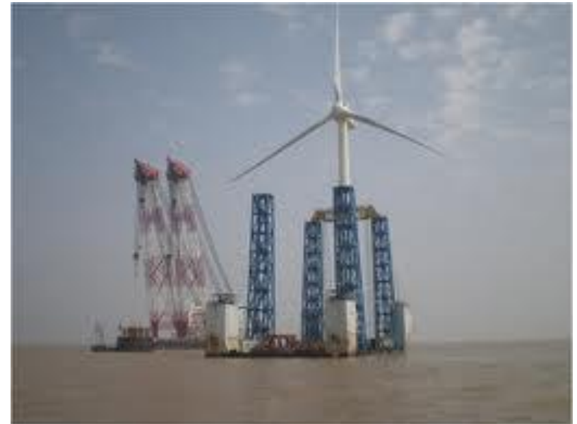
Rambiz installing WTG and tower complete at Beatrice Demonstrator
