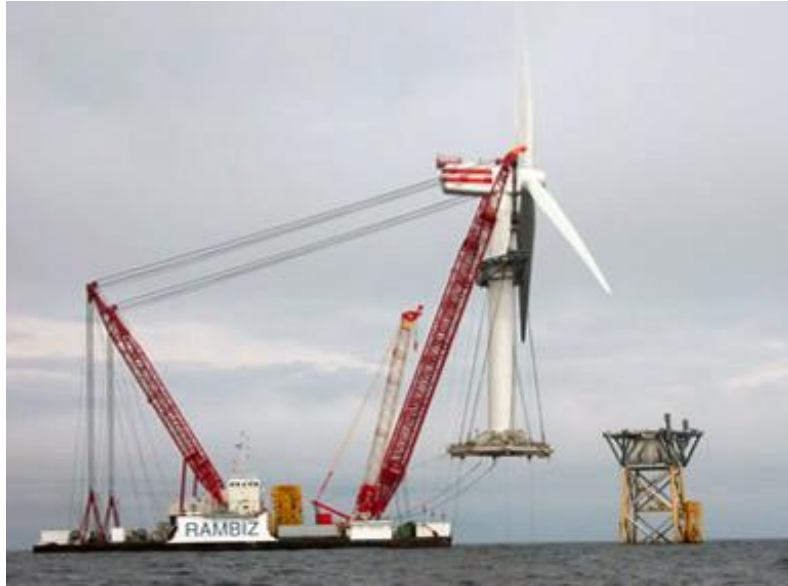
Rambiz installing WTG and tower complete at Beatrice Demonstrator
