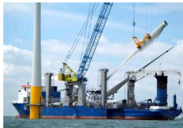
Leg-stabilised crane vessel
